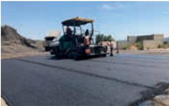
Warm Mix Asphalt at production temperatures below 120 °C. ASFALTMIN project
